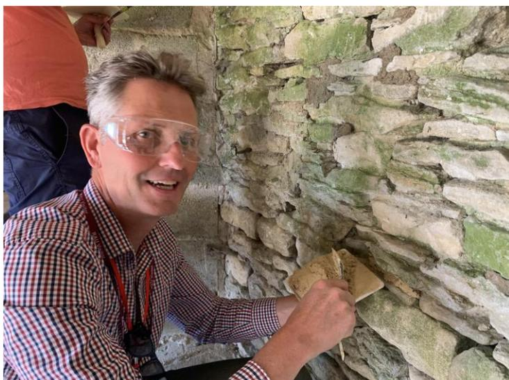
Stephen with trowel in hand practicing his re-pointing skills using quick lime putty mortar on an old rubble filled stone wall. (Quick lime is not to be confused with hydrated lime which builders add to cement mortar to improve workability).
